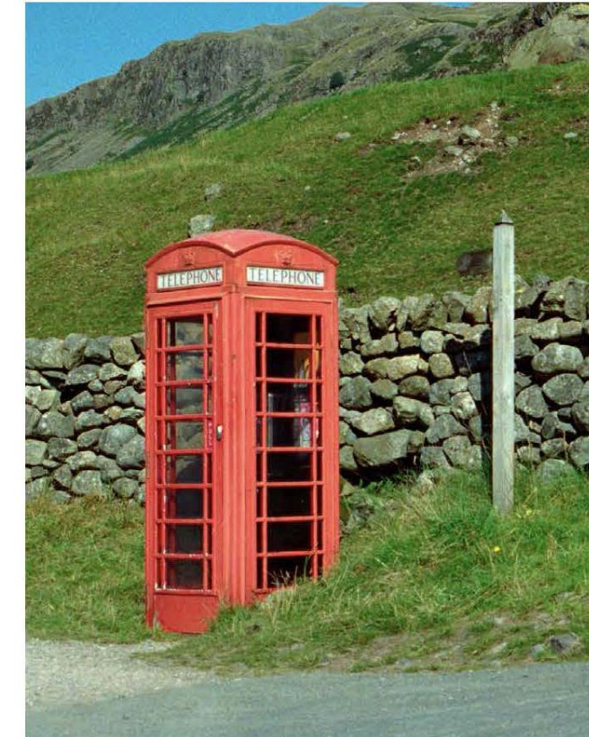
Figure 12 A Grade II listed K6 type telephone kiosk on the Eskdale Hardknott Pass, Cumbria. This type was designed in 1935 by Sir Giles Gilbert Scott and made by various contractors out of cast iron. The dramatic setting adds to the interest of this example.
